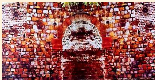
Remnant of wall of Delhi Jail
